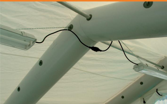
The inflatable arches are individually removable and connected mechanically to the covering fabric. Each inflatable arch features an inner tube and an outer layer.
